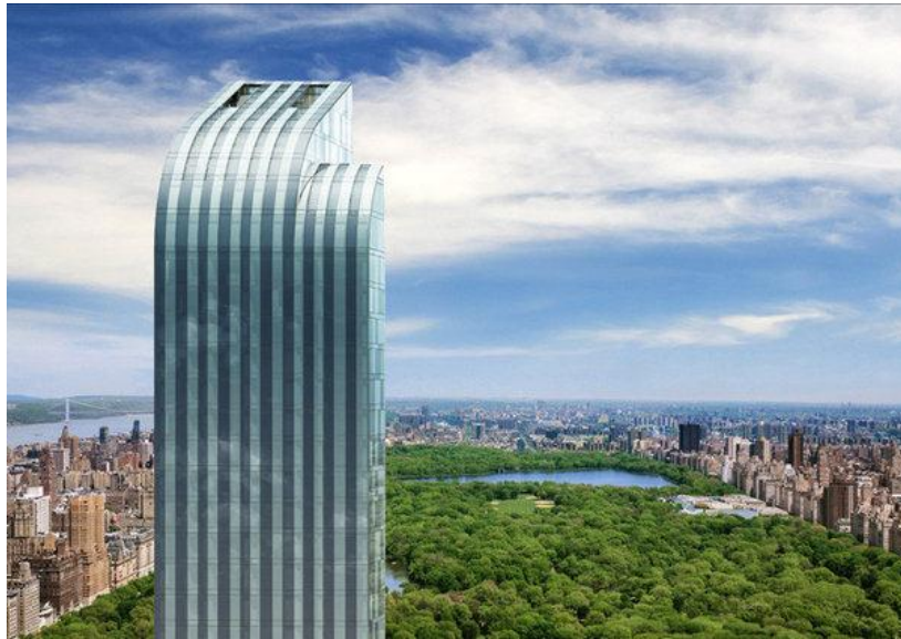
The One57 tower under construction in New York. (Extell Development Co. / May 21, 2012)
